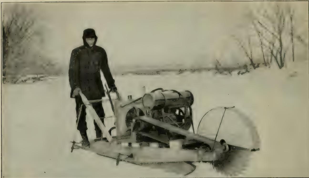
A SPEEDY ICE-CUTTING MACHINE
